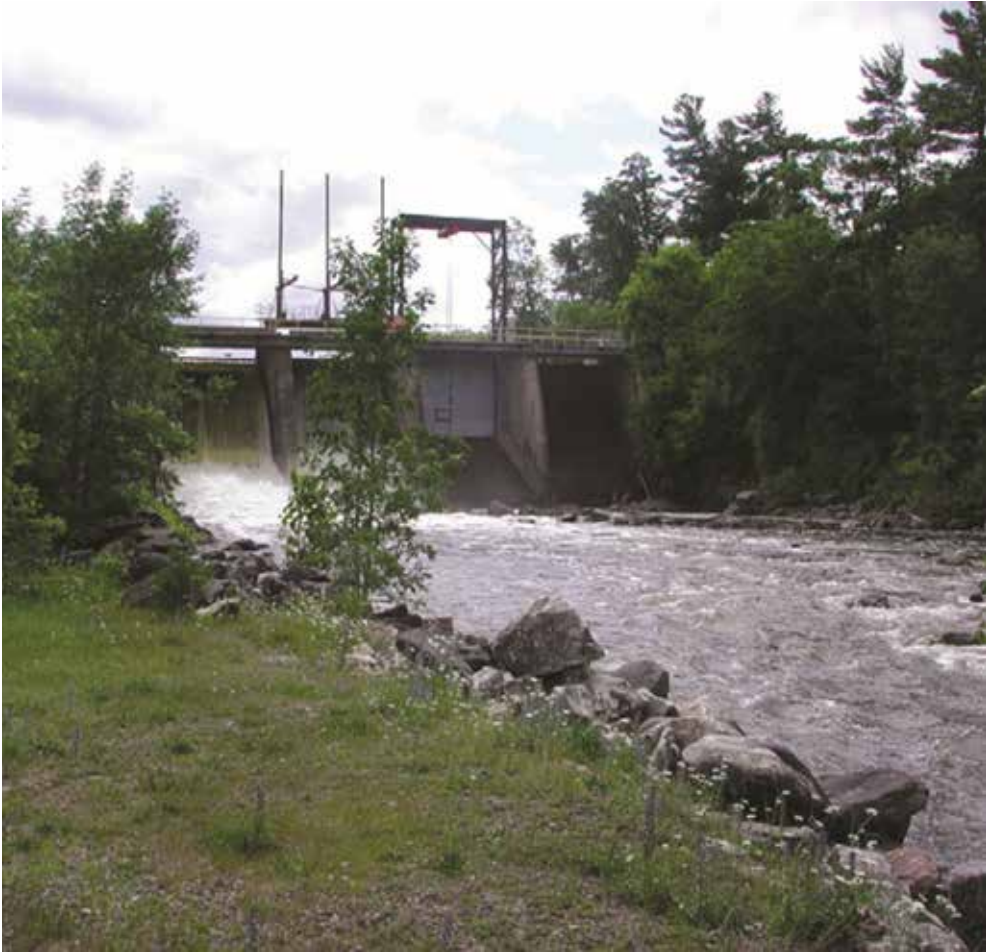
Figure 8 Run-of-River facility on the Bonnechere River
