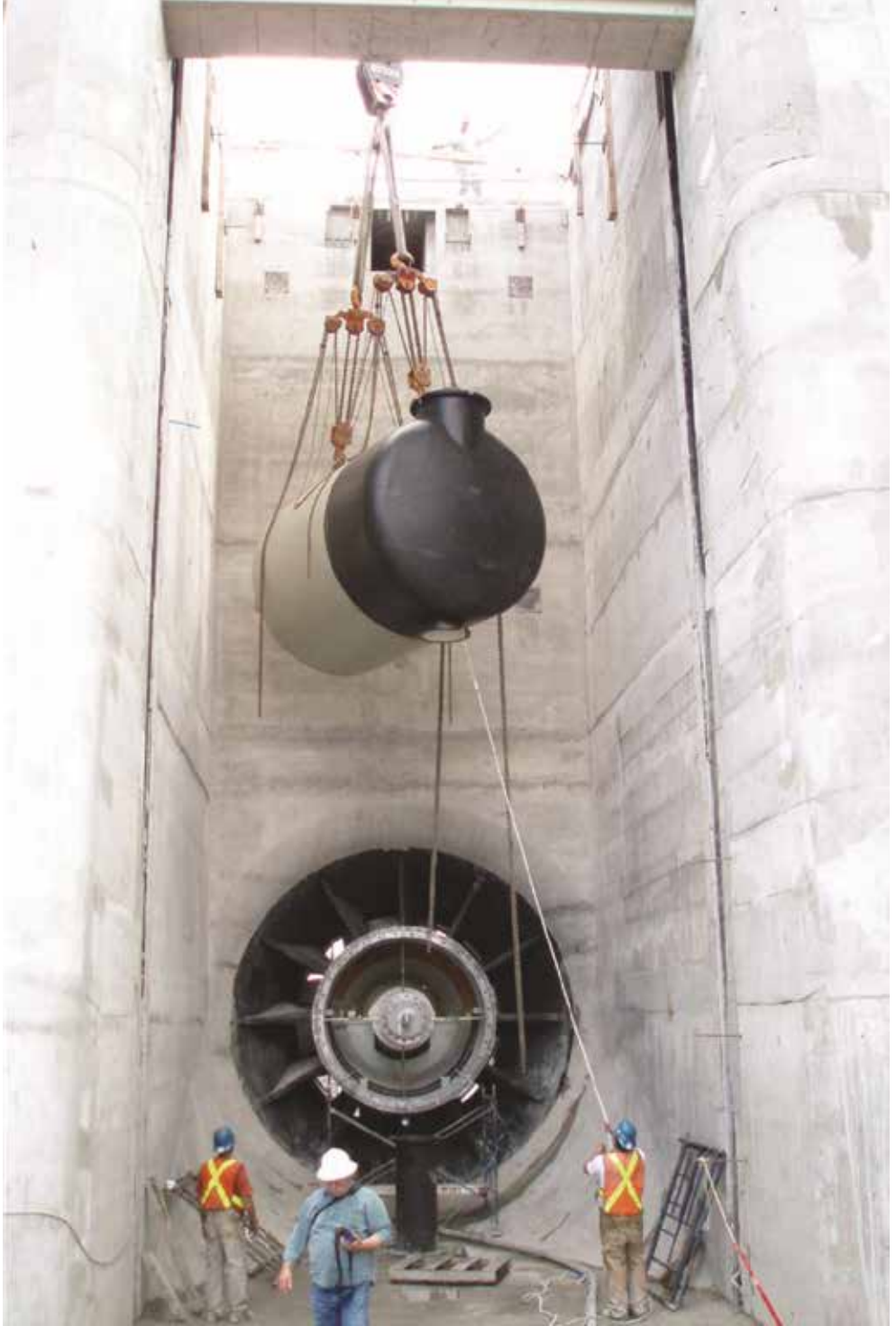
Figure 1 Construction phase of community waterpower development.
