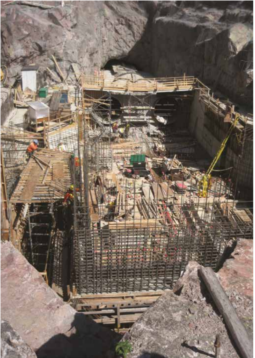
Figure 18 Construction phase at Umbata Falls, Wawa
