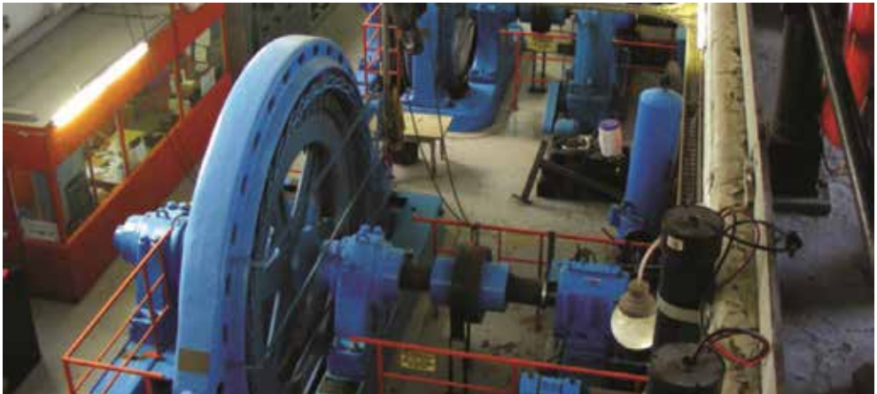
Figure 7 View inside a powerhouse
