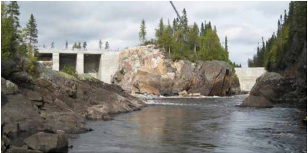
Figure 11 Run-of-river facility under construction at Umbata Falls
