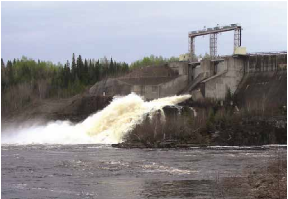
Figure 22 Matagami River Generating Station
