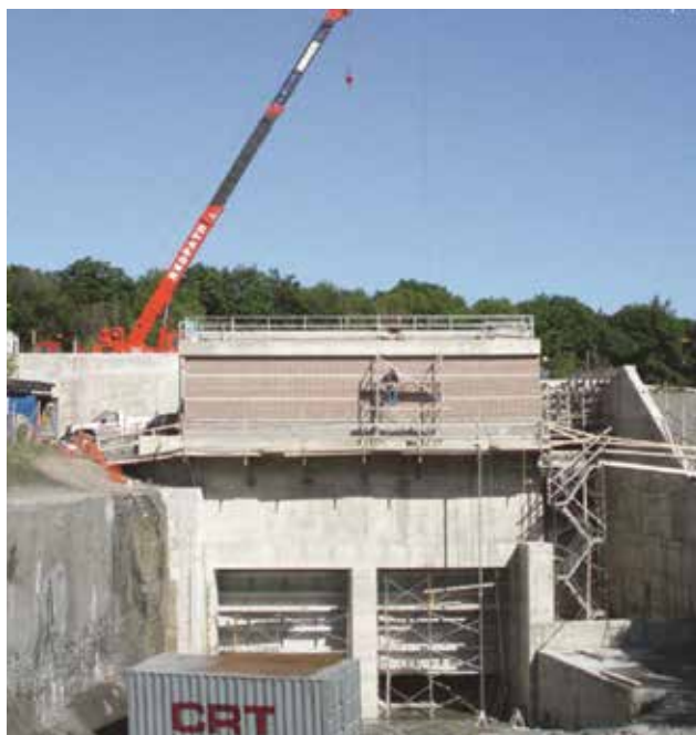
Figure 4 Construction phase of community waterpower development.
