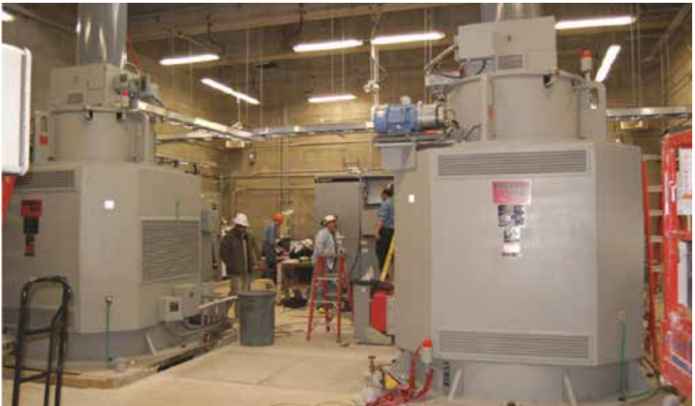
Figure 23 Generator room of a community waterpower facility under construction
