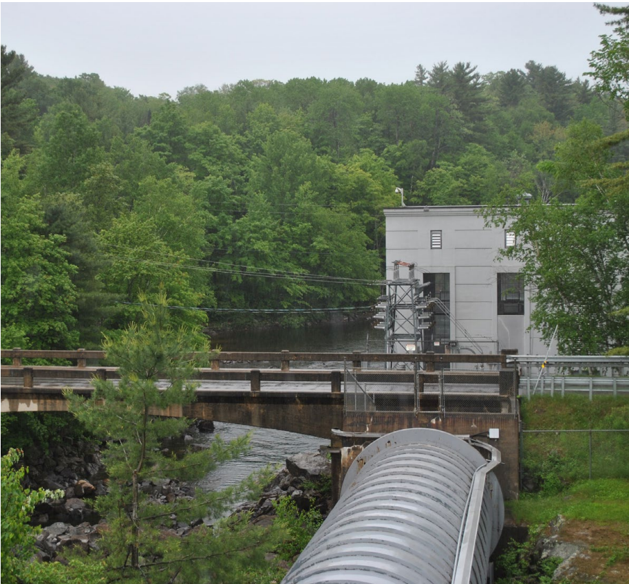
Figure 15: Example of Run-of-River with modified peaking facility. Matthais Generating Station (2.96 MW), located in Muskoka Ontario - Orillia Power Corp.
