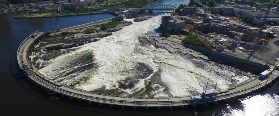
Figure 4: Chaudière Falls (29 MW) located in the City of Ottawa - Hydro Ottawa
