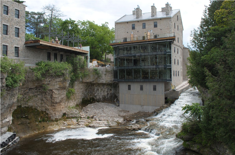
Figure 23: Elora Generating Station (1 MW) - Shawman Power Corp.
