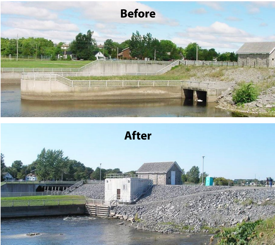
Figure 10: Small Waterpower Application at McLeod Dam, Quinte Conservation
