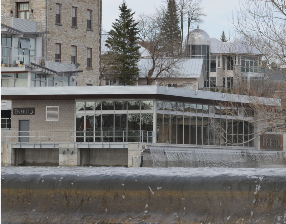
Figure 22: Enerdu Generating Station (1 MW) located in Almonte, Ontario - Enerdu Power Systems Ltd.
