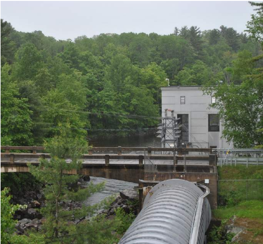
Figure 18: Example of Run-of-River with modified peaking facility. Matthais Generating Station (2.96 MW), located in Muskoka Ontario - Orillia Power Corp.
