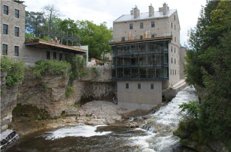
Figure 26: Elora Generating Station (1 MW) - Shawman Power Corp.
