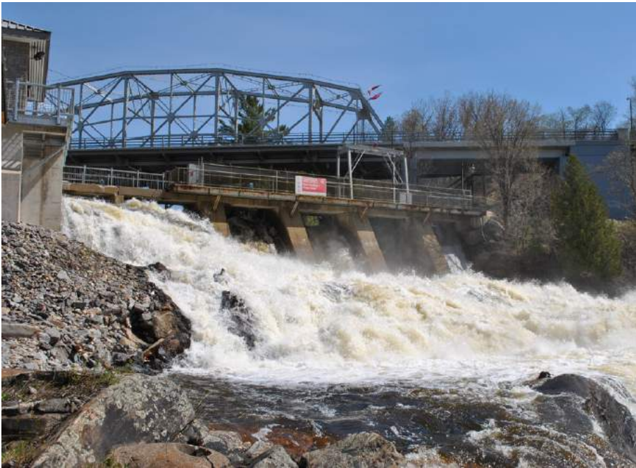
Figure 25: Bracebridge Falls Generating Station (2.6 MW) - Bracebridge Generation Ltd.
