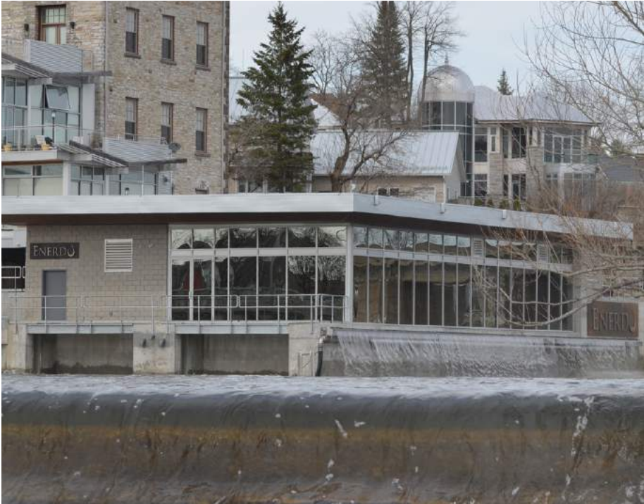
Figure 24: Enerdu Generating Station (1 MW) located in Almonte, Ontario - Enerdu Power Systems Ltd.
