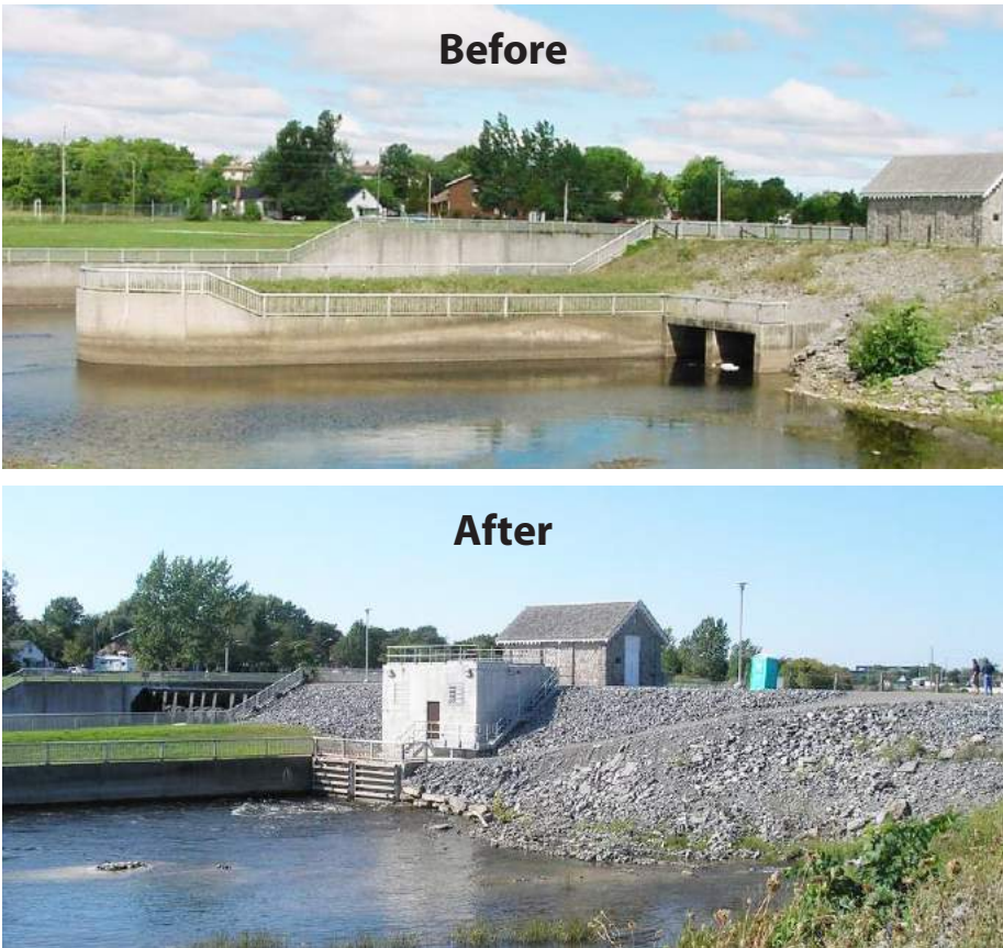
Figure 10: Small Waterpower Application at McLeod Dam, Quinte Conservation
