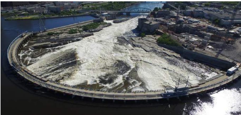
Figure 4: Chaudière Falls (29 MW) located in the City of Ottawa - Hydro Ottawa
